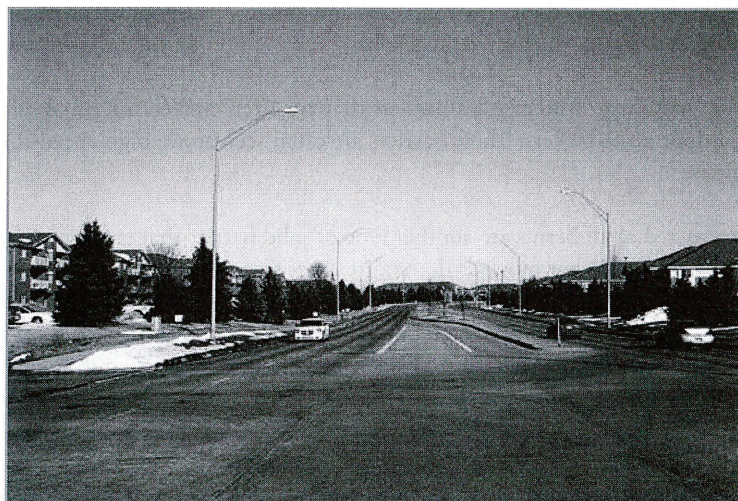
A single row of trees will not provide noticeable noise reduction. At best they will provide a visual screen between residents and the noise source.
